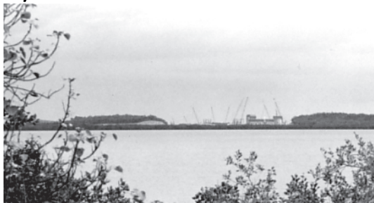
Highly visible LNG plant viewed from across the harbour.
